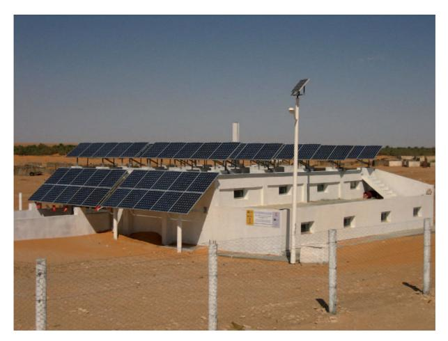
Figure 23: A 2.1 m<sup>3</sup>/h nominal capacity brackish water PV-RO plant in Tunisia, installed by the Canary Island Institute of Technology, Spain.
