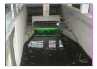
Figure 6-13 UV disinfection and chlorination
