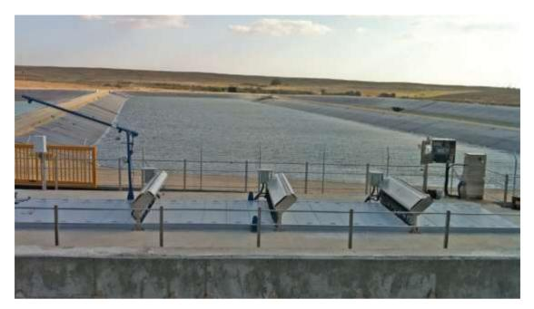
FIGURE 4-7 UV DISINFECTION SYSTEM (WITH EFFLUENT PONDS BEHIND)
