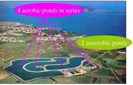
Waste Stabilization Ponds system to secondary and tertiary treatment 20.000 PE in Mezé (France)
