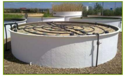
Filter substrate thickness: 0.6 m
