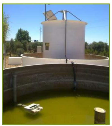
Filter substrate thickness: 1.5 m
