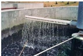
Also known as percolating filters, are the most traditional method of biofilm process used for the biological treatment of wastewater.
