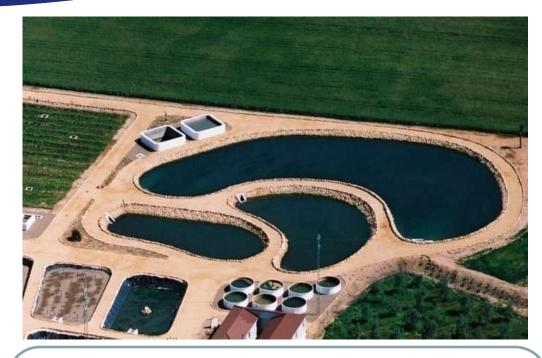
It is made up of several lagoons connected in series. Their depth is gradually reduced and they alternately present conditions of absence or presence of oxygen. They reproduce the water selfpurification process that is found in natural water courses
