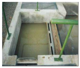
Static grease chamber with a superficial system for grease removal
