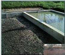
Sewage filtration through beds using peat as filtering medium. A series of physicalchemical and microbiological properties which make it especially suitable for urban liquid waste purification.
