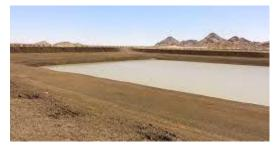
**Cisterns, hafirs and dams are indigenous methods** widely used in arid and semi-arid areas for runoff water harvesting. A large number of cisterns existing in the region are linked with the Roman period. **Cisterns** are underground structures excavated in the frail rock to provide a water storing capacity that could range from 100 m3 to 3000 m3 (ICRISAT, 1999). The structure consists
