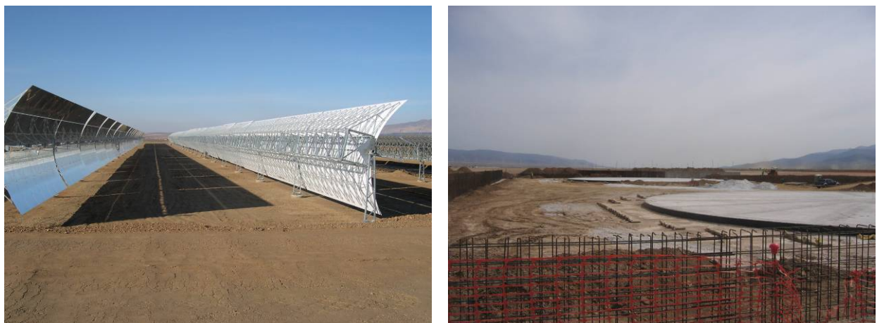
Figure 1-16: Parabolic trough collectors and foundations for the molten salt tanks of ANDASOL 1.
