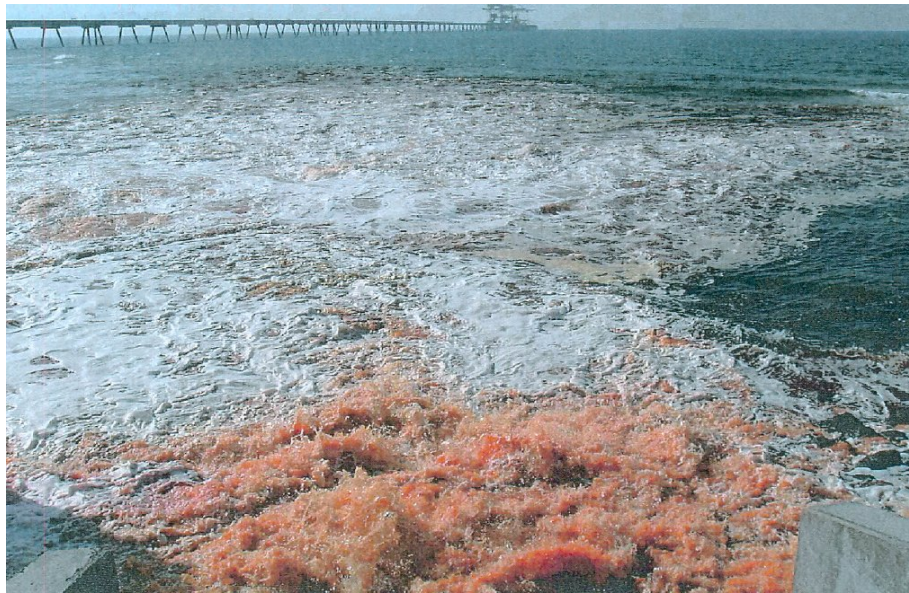
Figure 6-12: Red brines containing ferric sulphate from filter backwash at Ashkelon RO desalination plant; backwash with 6,500 m 3 in 10-15 minutes every hour. Photo: Rani Amir, Director of the Marine and Coastal Environment Division of the Ministry of the Environment, presented by Iris Safrai, Ministry of the Environment, at the EDS Conference on Desalination and the Environment, Halkidiki, Greece, April 2007.
