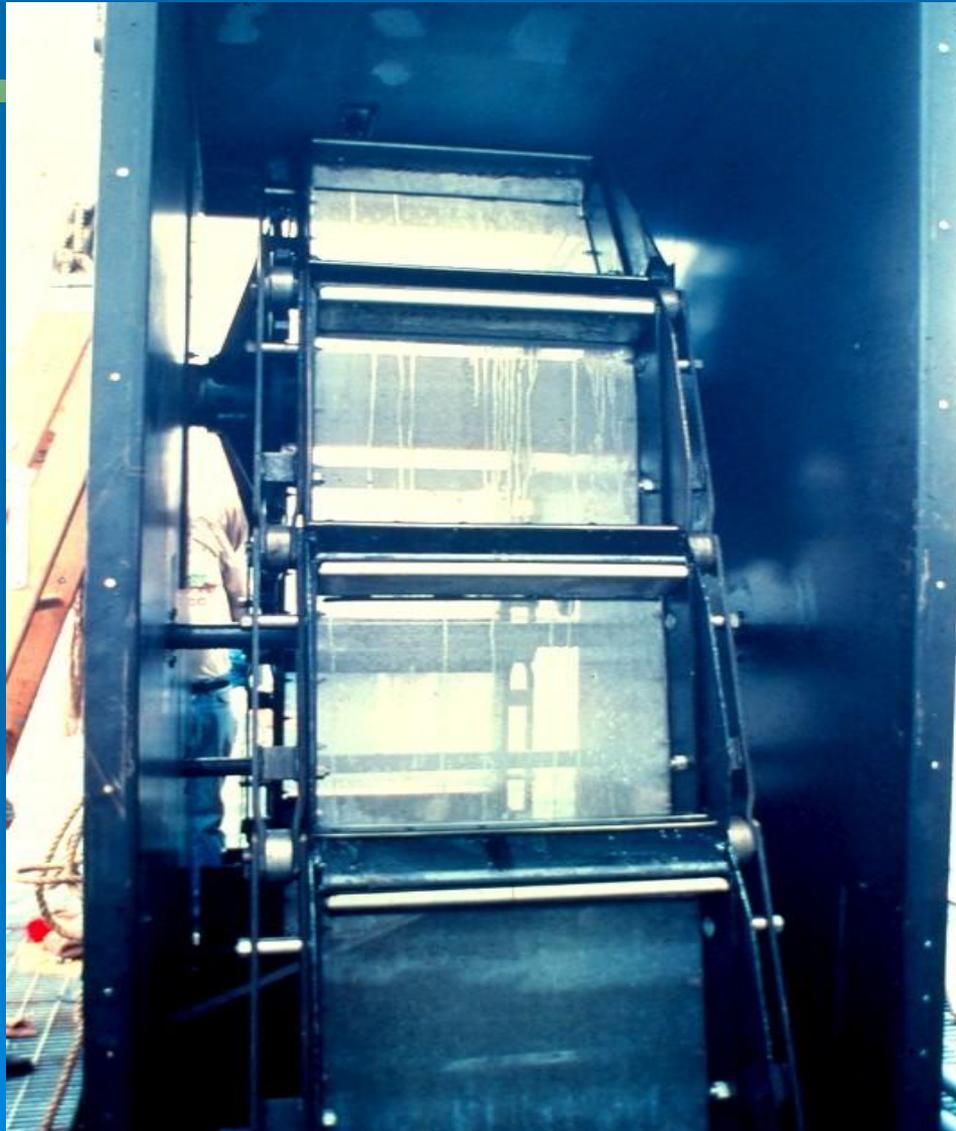
500  $\mu$ Travelling Band Micro-screens – Tampa Bay Water SWRPO Plant Intake
