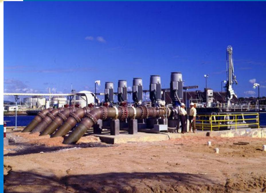
**Near-shore Intake – Point Lisas Desalination Plant, Trinidad**
