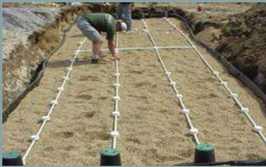
Shallow beds (0.6-1.1 m deep), equipped with a surface distribution system for the sewage and a drainage piping to collect the treated effluent at the bottom of the filter.
