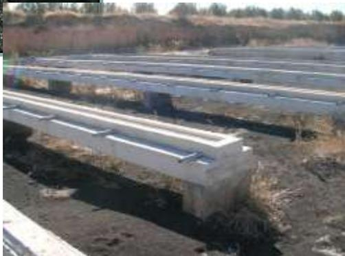
Sewage filtration through beds using peat as filtering medium. A series of physical-chemical and microbiological properties which make it especially suitable for urban liquid waste purification.
