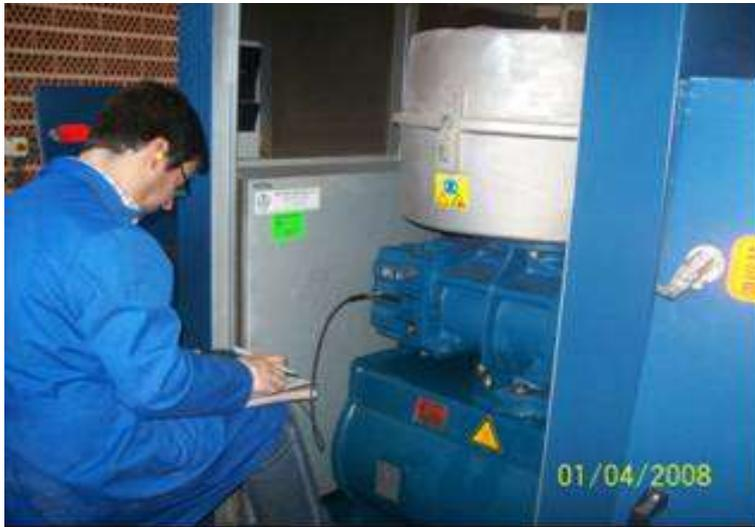
Predictive maintenance by measuring vibrations of a blower
