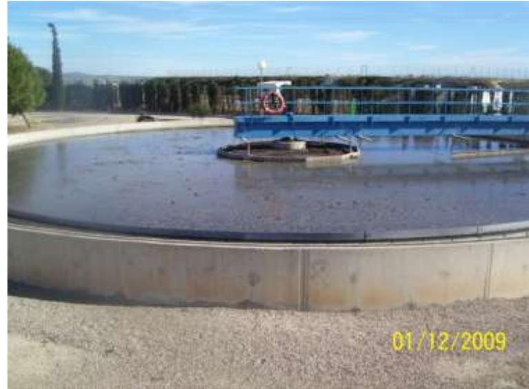
Filamentous foaming in a biological reactor and secondary sedimentation tank.
