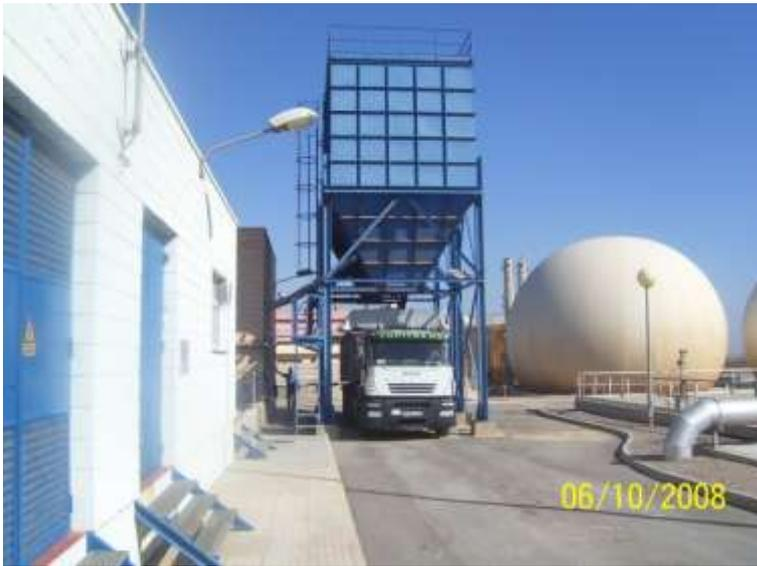
Load of sludge for transport to composting plant
