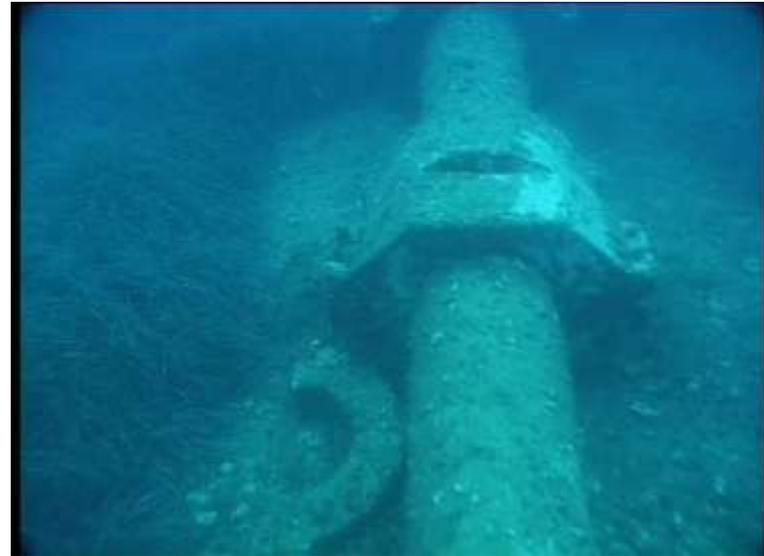
Drawing of the submarine outfall of San Pedro (Murcia) and photograph with broken ballasts
