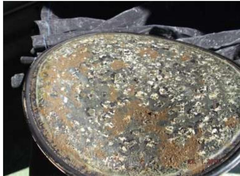
Checking the operation off the air diffusers and detail of a clogged one
