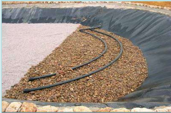
Flux ZHA horizontal subsurface
