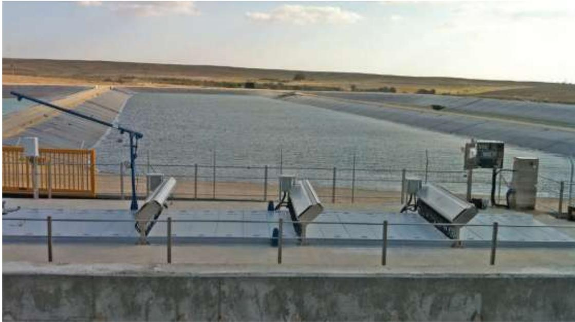
FIGURE 4-7 UV DISINFECTION SYSTEM (WITH EFFLUENT PONDS BEHIND)
