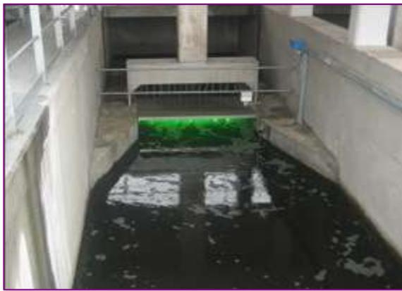
Figure 6-13 UV disinfection and chlorination
