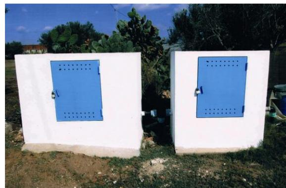
Water meters in a protective box at each farm gate
