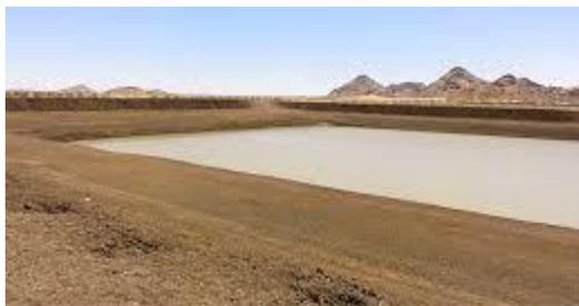
**Cisterns, hafirs and dams are indigenous methods** widely used in arid and semi-arid areas for runoff water harvesting. A large number of cisterns existing in the region are linked with the Roman period. **Cisterns** are underground structures excavated in the frail rock to provide a water storing capacity that could range from 100 m<sup>3</sup> to 3000 m<sup>3</sup> (ICRISAT, 1999). The structure consists of channels to collect
