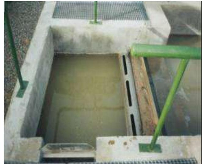
Static grease chamber with a superficial system for grease removal
