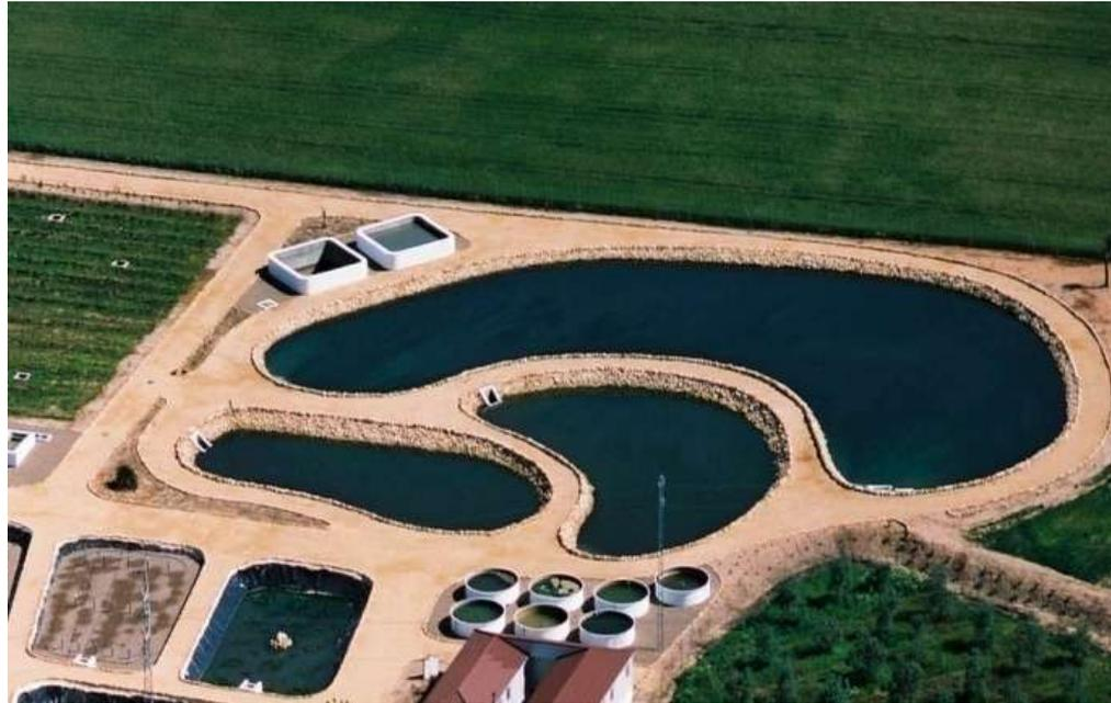
It is made up of several lagoons connected in series. Their depth is gradually reduced and they alternately present conditions of absence or presence of oxygen. They reproduce the water self-purification process that is found in natural water courses
