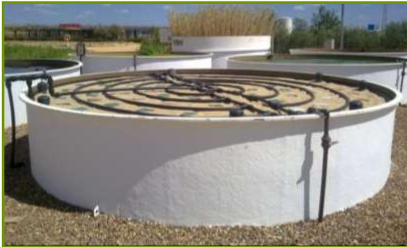
Filter substrate thickness: 0.6 m
