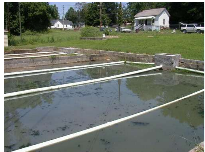
Overload in a Intermittent Sand Filter
