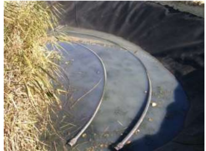
Clogging in Horizontal Constructed Wetland
