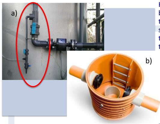
The sampling point will be realized through a tap if directly applied on the pipe (see image a for example) or a small tank (see image b for example).
