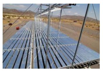
Fig. 8. Photo of the linear Fresnel concentrator erected at the PSA
