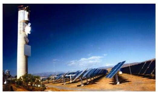
*Fig. 3. The CESA-I facility seen from the East with heliostat rows focusing on the medium-height test level (60 m.)*
