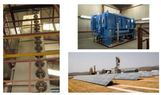
Fig. 17. PSA SOL-14 MED Plant (left), double-effect LiBr-H2O absorption heat pump (upper right) and 500-m2 CPC solar collector field (bottom right)
