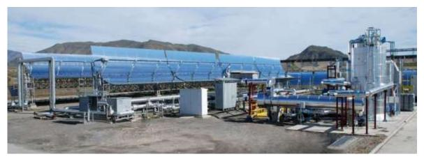
Fig. 7. View of the pressurized gas test loop connected to a molten-salt thermal energy storage
