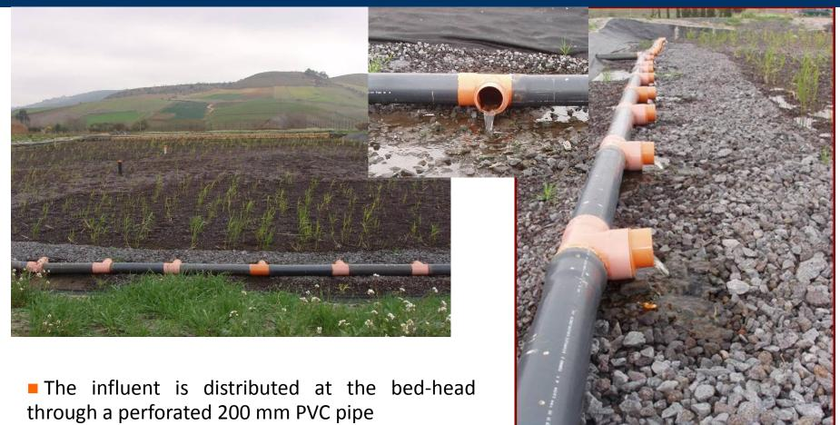
coarser rock with larger void spaces and a higher hydraulic conductivity was used at inlet zone to ensure rapid infiltration, and at outlet zone to favorite flow collection
