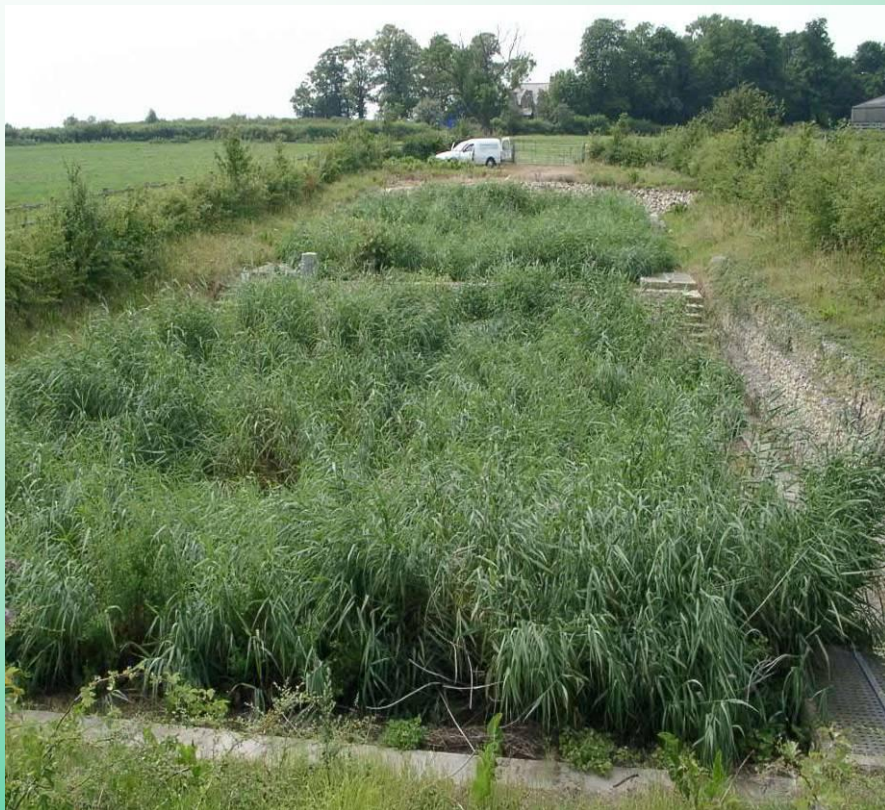
Sub-surface flow reed bed in Saxby, England (Severn Trent Water), two beds in series.
