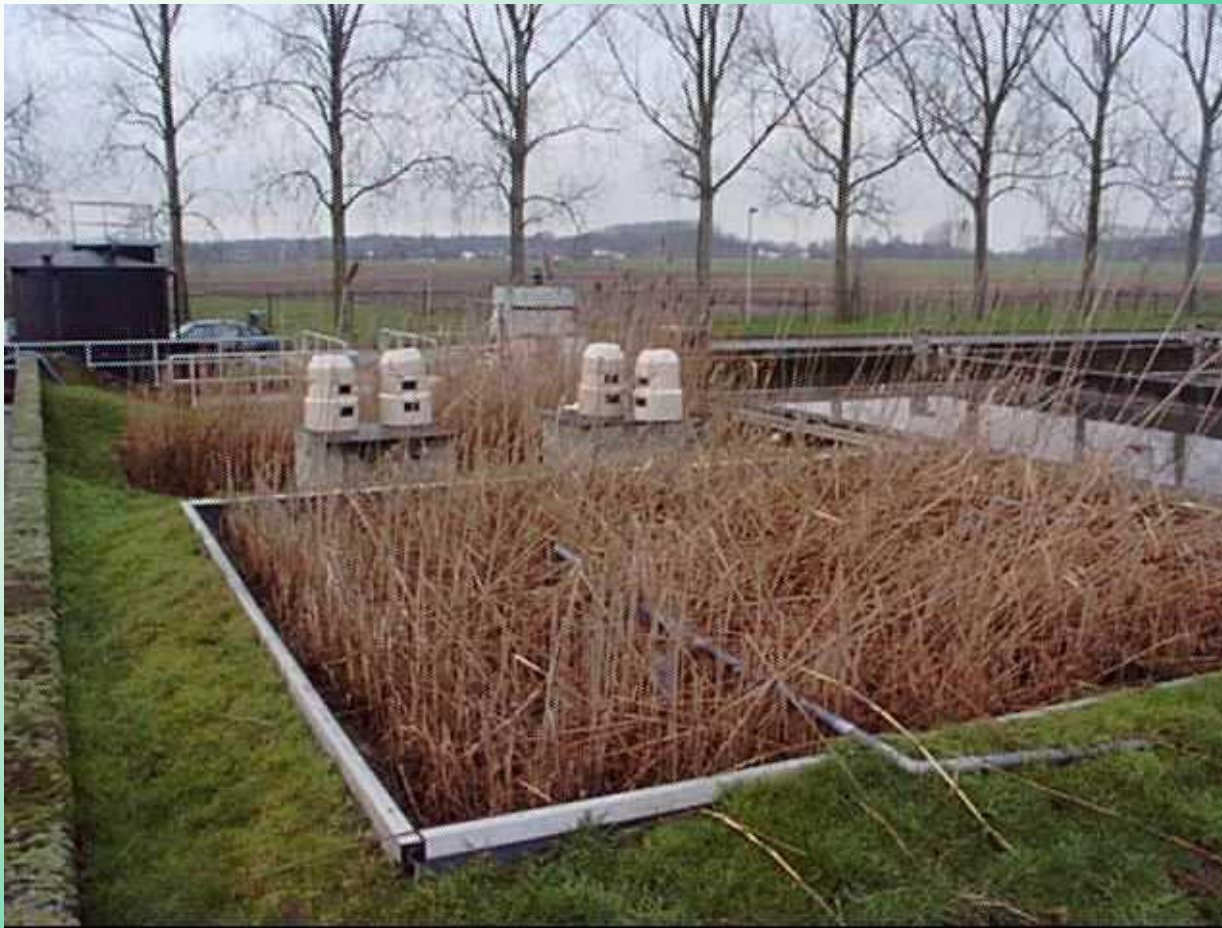
Experimental CW in Aartselaar (Belgium), Aquafin Ltd. Foreground: two parallel VF beds (first stage). Background: two parallel HSSF beds (second stage).
