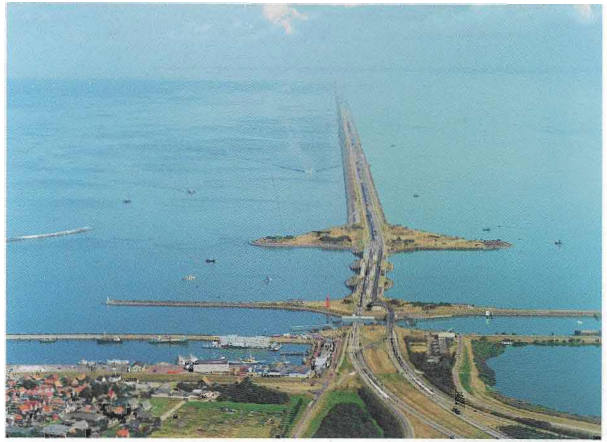
Figure 4.8 The 32 km long main dam (Afsluitdijk). Left: Wadden Sea (salt water), right: Lake IJssel (fresh water)
