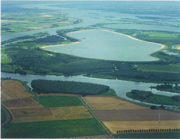
Figure 5.7 Reservoirs for drinking water in the Biesbosch
