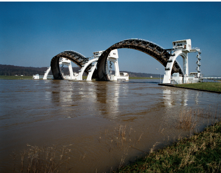
Weir in the Neder-Rijn at Driel.
