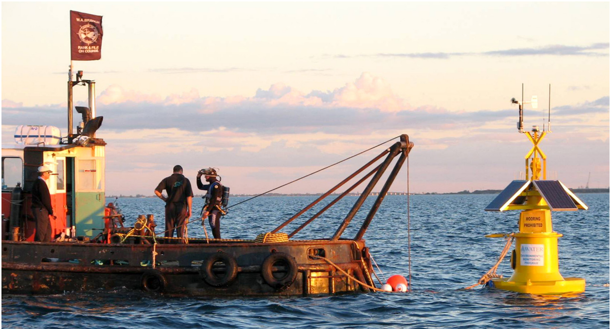
Figure 4: Deployment of a real time monitoring buoy for the Perth seawater desalination plant (by courtesy of 360 Environmental, Environmental Management Consultants, Australia).
