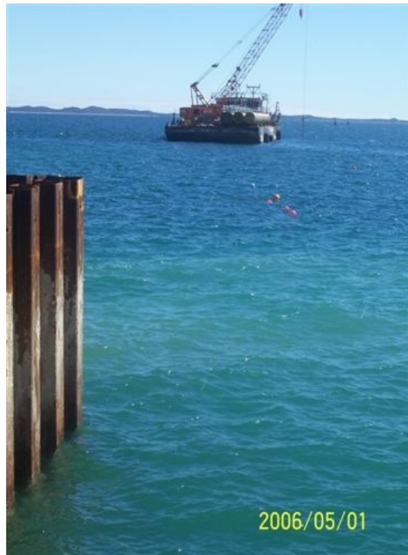
Figure 6: Construction of a sheet pile trench for the Perth seawater desalination plant with minor plume development (by courtesy of Water Corporation of Western Australia).
