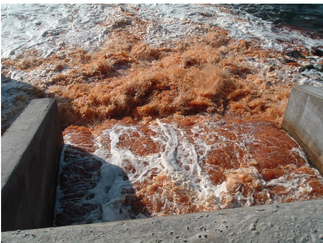
Figure 11: Periodic discharge of filter backwash water from the Ashkelon SWRO plant in Israel (courtesy of Rani Amir, Director of the Marine and Coastal Environment Division, Israel Ministry of the Environment).
