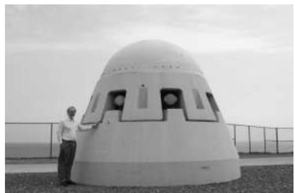
Figure 22: Boston outfall during installation in 1998. *Left*: View into tunnel section (16 km with 8 m diameter). *Right*: One out of 55 riser caps with eight outlets each in rosette-like configuration (Roberts and Snyder, 1993)
