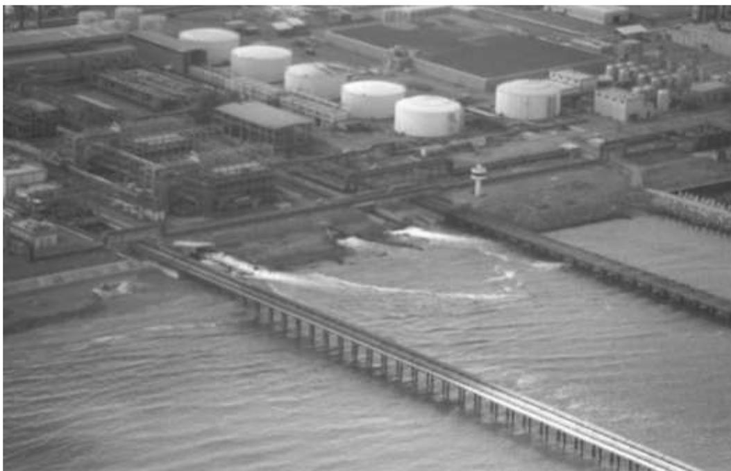
Figure 1: Al Ghubrah desalination plant (largest in Oman, capacity 191,000 m<sup>3</sup>/d): Brine discharge through an open channel at the coast into the Gulf of Oman (photo: H.H. Al-Barwani)
