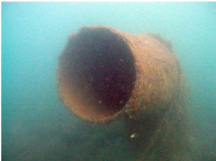
Figure 112: Outfall diffuser for discharge of brine (file photo: HMR Consultants)
