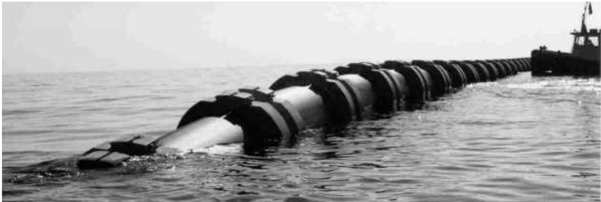
Figure 21: Antalya wastewater outfall (Turkey) during installation in 1997. *Top*: Diffuser section assembling on shore. *Down*: Feeder section ( $L_F = 5$  km, HDPE pipe,  $D = 1600$  mm) while sinking with attached concrete weights on the seabed (PipeLife Company)
