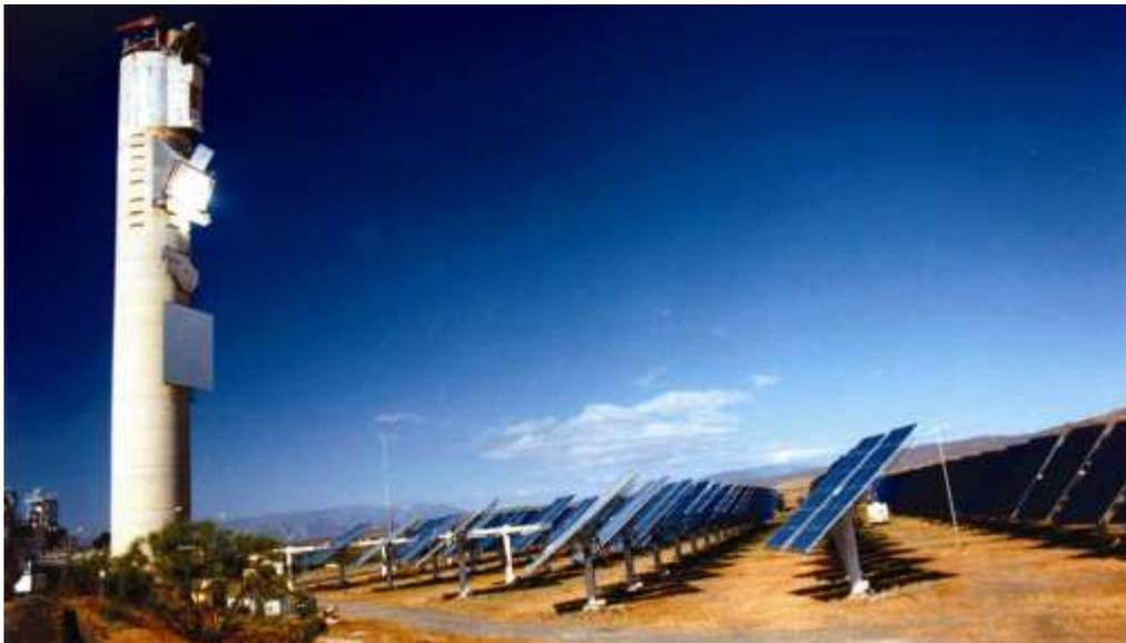
*Fig. 3. The CESA-1 facility seen from the East with heliostat rows focusing on the medium-height test level (60 m.)*
