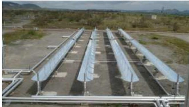
*Fig. 19. NEP PolyTrough 1200 solar field*
