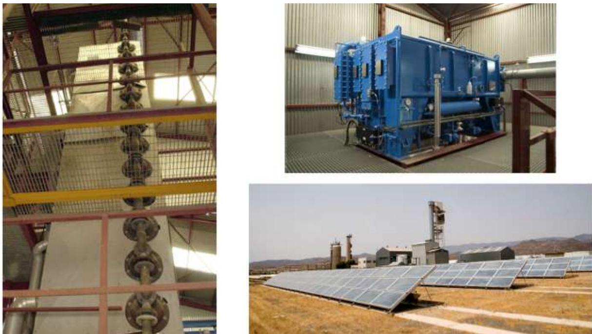
*Fig. 17. PSA SOL-14 MED Plant (left), double-effect LiBr-H<sub>2</sub>O absorption heat pump (upper right) and 500-m<sup>2</sup> CPC solar collector field (bottom right)*
