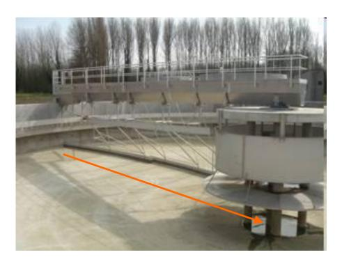
Circular settler (empty in the picture to show the internal structure): Bridge travels around and pushes accumulated sludge to central evacuation pipe
